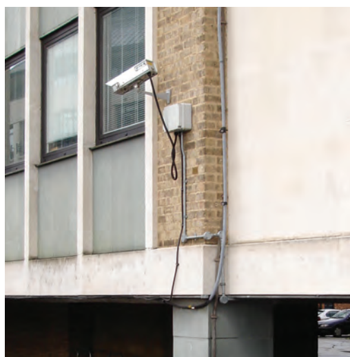
Figure 65. Conventional down-conductor separation distance problem.
