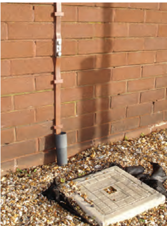
Figure 51. Typical down-conductor connectors.
