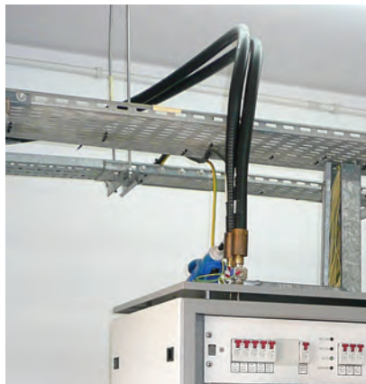
Figure 113. Incoming antenna circuits require protection.
