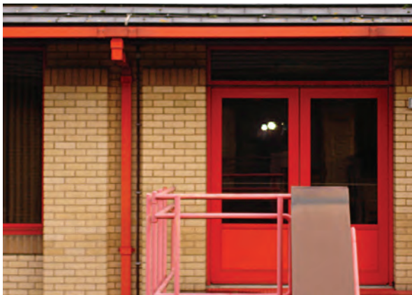
Figure 54. Example of poorly located a down-conductor.
