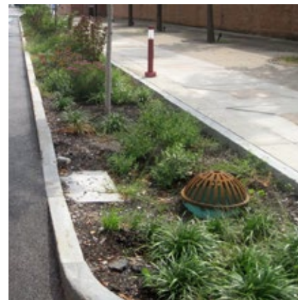
The overflow drain is placed in the flow path of water entering the practice.
