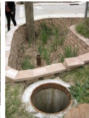
Figure 4-27. To facilitate maintenance, an observation well is installed next to a bioretention area in Houston, TX.
