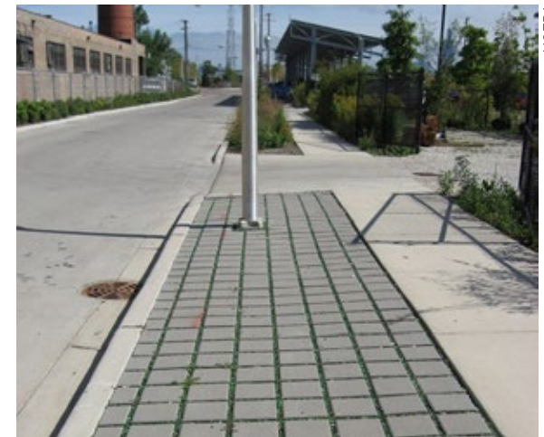
Figure 4-32. Tumbled green glass fills the spaces between permeable pavers in a sidewalk area in Chicago, IL.
