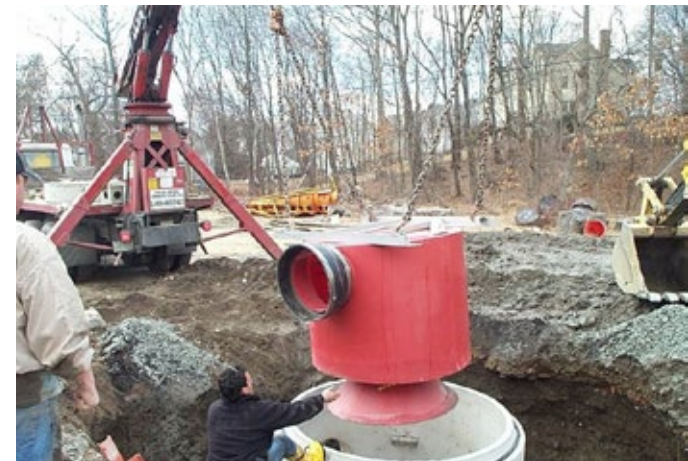
Vortex separator being installed.
