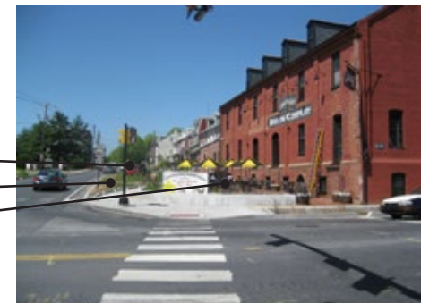
Figure 2-16. A roadway was reconfigured to replace a turn lane with green infrastructure practices in Lancaster, PA.
