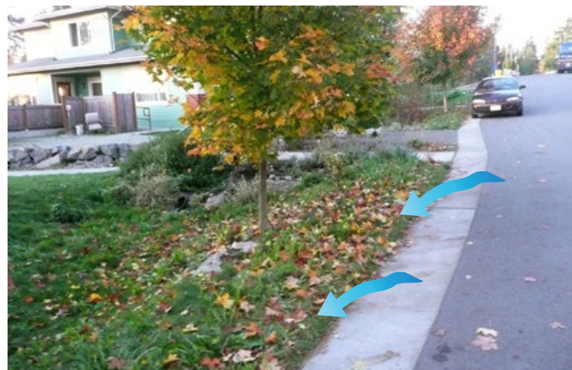
Figure 4-12. A sloped concrete band along a road evenly distributes stormwater to an adjacent vegetative swale in Seattle, WA.
