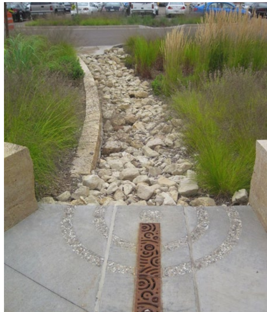
A sediment forebay provides pretreatment for a rain garden in Maplewood, MN.
