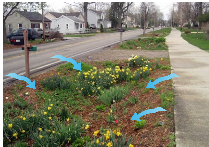
Figure 4-10. A curbless street allows sheetflow stormwater runoff to enter the vegetated swale in Lansing, MI.
