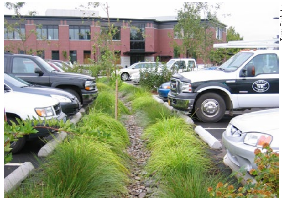
Figure 2-14. In this parking lot the median space between facing parking stalls includes a bioretention area.
