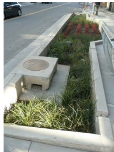
Figure 4-21. Raised overflow drain allows a design volume of stormwater to collect in a bioretention area in Portland, OR.
