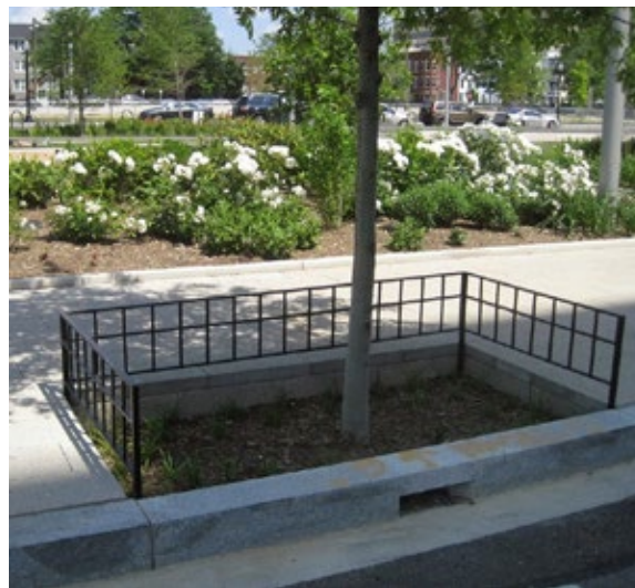
Figure 4-35. Short fencing protects pedestrians from stepping into this stormwater tree box in Washington, DC.
