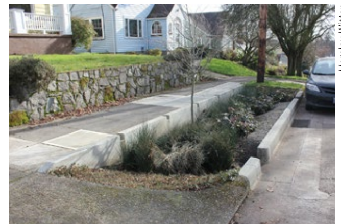
Curb cuts in the sidewalk and street allow for runoff to flow into this stormwater planter in Portland, OR.
