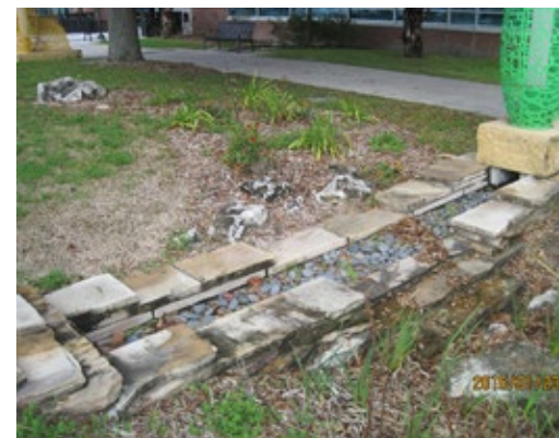
Figure 4-16. A piled stone weir/gravel filter combination slows the water flowing through this bioretention feature in Gainesville, FL.
