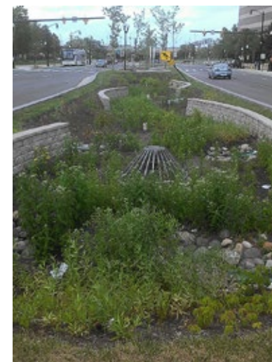
Figure 4-22. Beehive overflow grate prevents debris from entering the overflow structure in a roadside bioswale in Arlington, VA.
