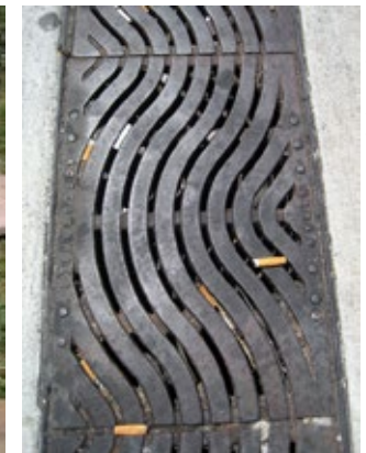
Figure 4-28. The small spaces in this grate are clogged with cigarette butts, which block drainage and are difficult to remove.
