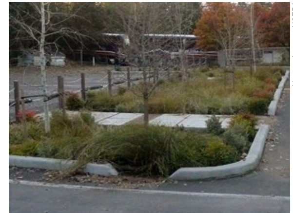
Figure 4-30. Walkway built across vegetated swale to allow users to access their cars in Portland, OR.
