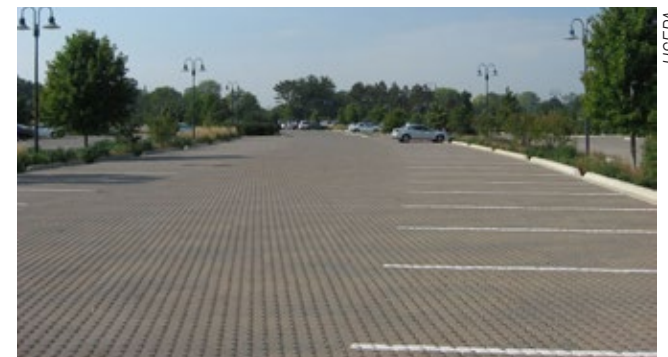
Permeable interlocking concrete pavement, Chicago, IL.
