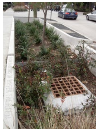
Figure 4-19. Raised overflow structure in a bioretention feature in Houston, TX.
