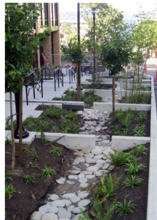
Figure 4-18. Concrete check dams with splashpads slow flow velocities along a steep slope in Seattle, WA.
