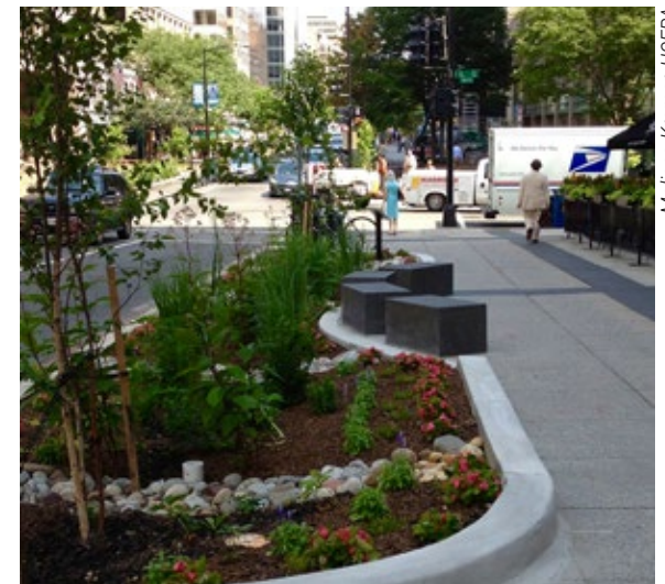
Figure 4-36. Seating adjacent to a bioretention unit provides an amenity for passersby and also serves as a barrier in Washington, DC.
