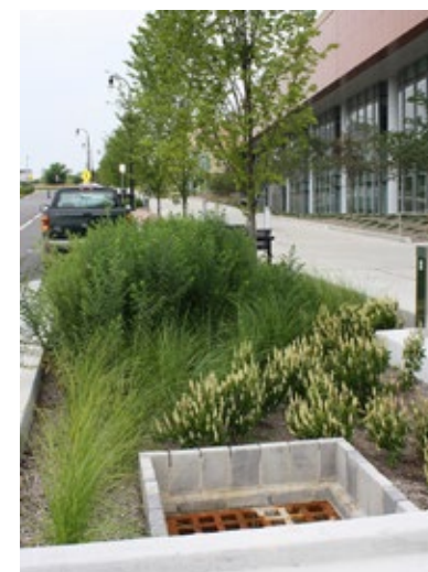
Figure 4-20. Concrete band constructed around the outflow allows ponding in Nashville, TN.
