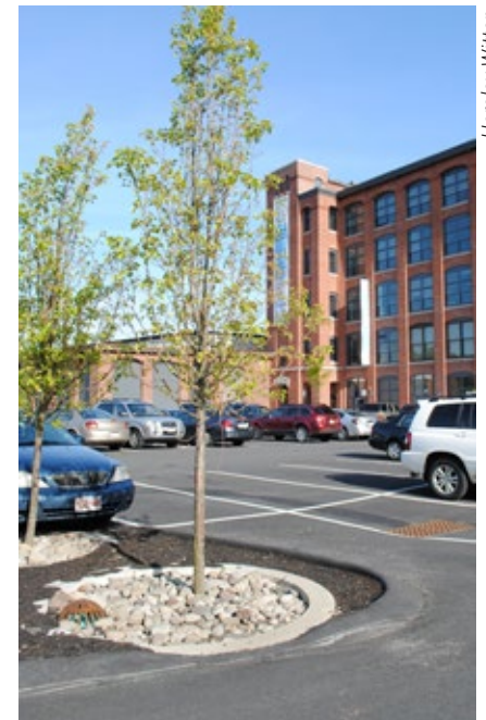
A tree pit captures runoff in a parking lot in Lawrence, KS.
