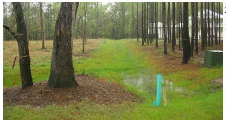
Infiltration trench with grass cover.
