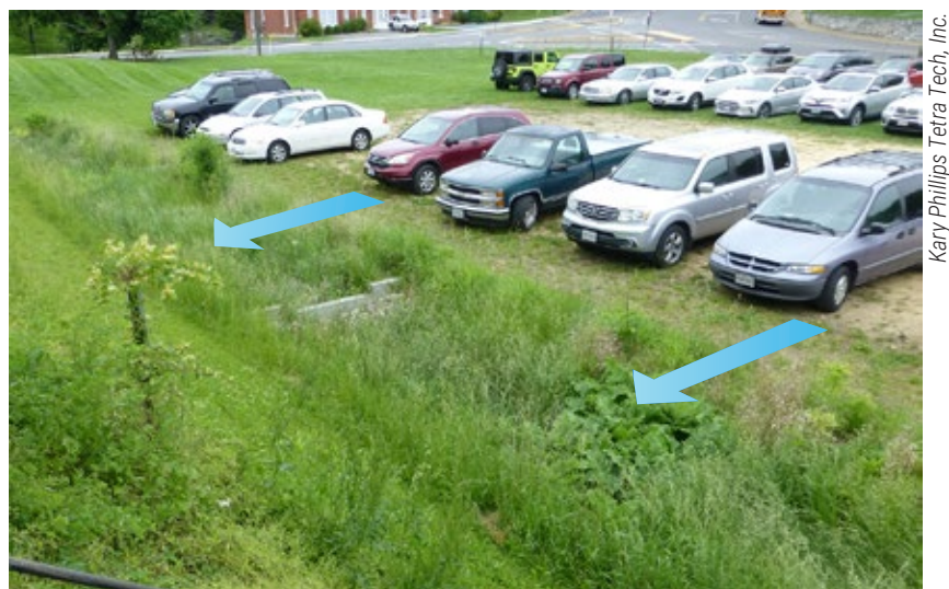
Figure 4-11. A curbless grassed and gravel parking lot allows sheetflow stormwater runoff to enter a vegetated swale in Staunton, VA.
