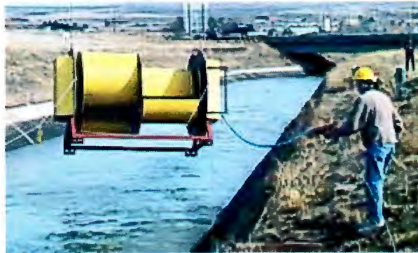
Roza Canal: Testing innovative hydrokinetic devices
