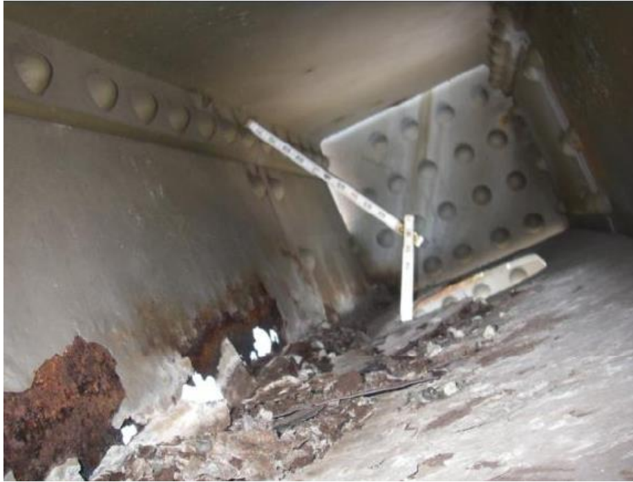
Figure 33. Photo. Inside of built-up box member.
