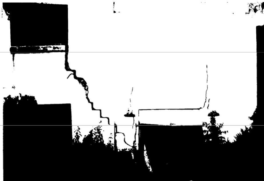
b. Diagonal and vertical cracks
