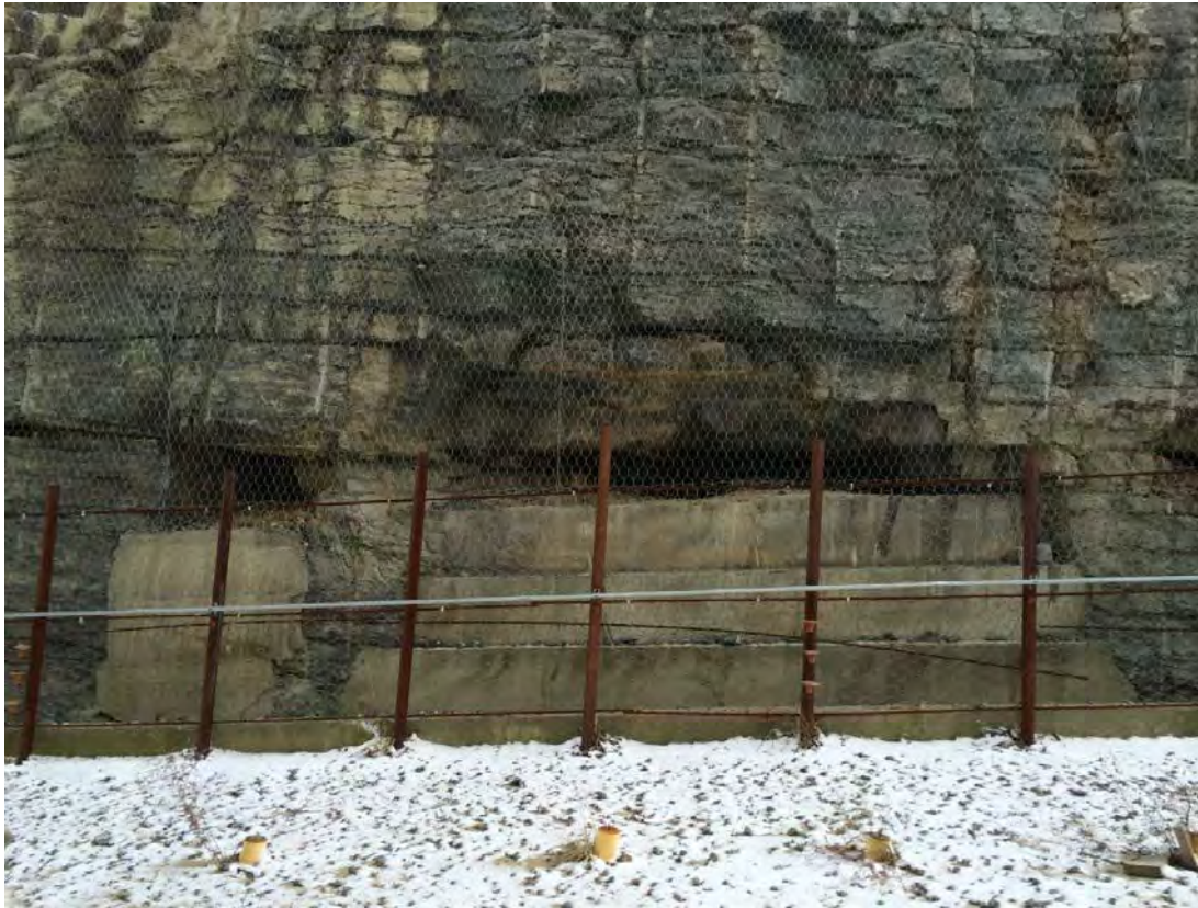
Figure 47. View of Karst Feature at Base of Presplit with Concrete Added at Cave Mouth.
