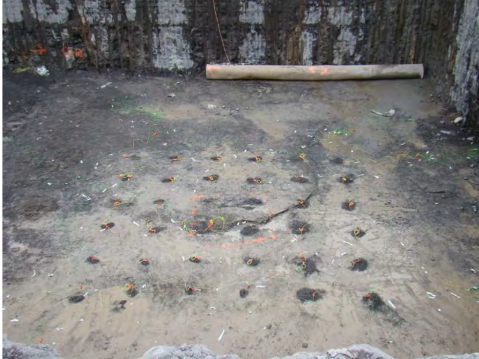
Figure 6. Sinking Shot Loaded and Hooked up for Excavating a Lock Monolith Foundation.
