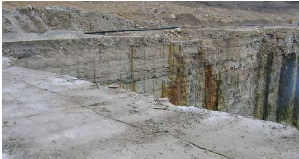
Figure 45. Tension Crack in Rock Mass after Presplit Blasting.
