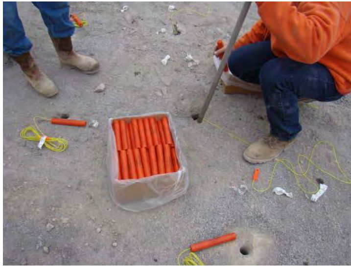
Figure 35. Primers with Caps Inserted Ready to Be Loaded into Blastholes.
