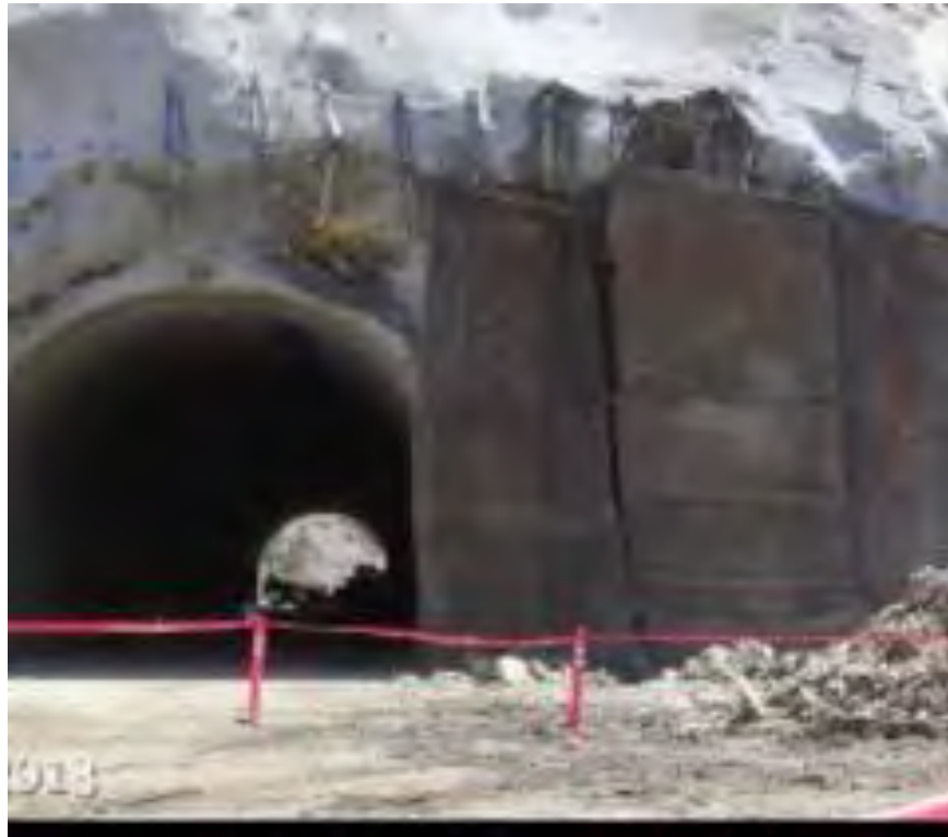
Figure 8. Wire Blasting Mats Protects Structures
