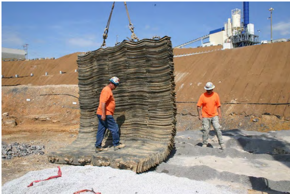
Figure 7. Rubber Blasting Mats Being Lowered onto Shot at Kentucky Lock.
