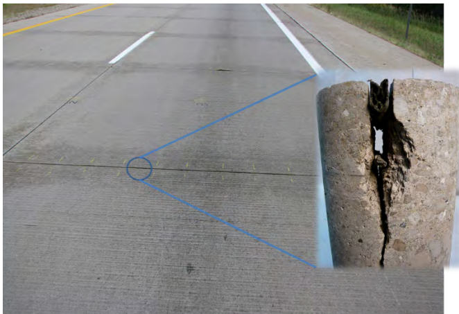
Figure 5. Joints on I-94 in Michigan showing surface "shadowing." Extracted core reveals high degree of damage below the surface in zone of high degree of saturation (courtesy Dr. Karl Peterson).
