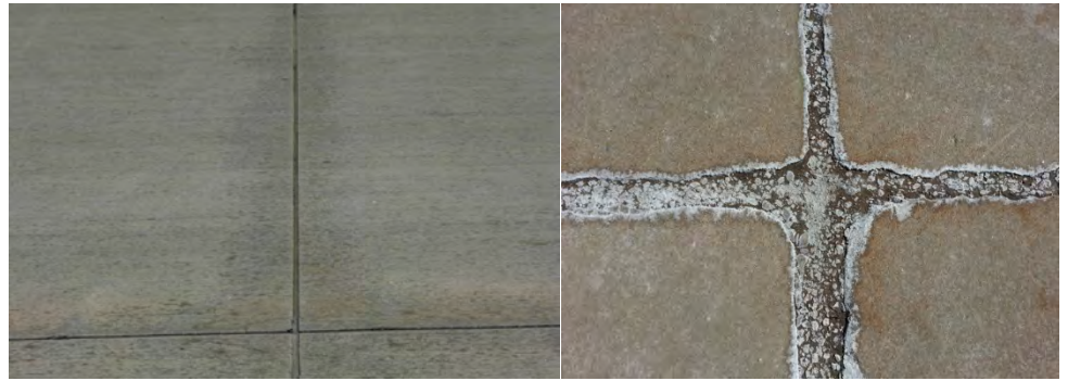
Figure 1. Joint “shadowing” (left) and eventual disintegration of concrete at joint (right).
