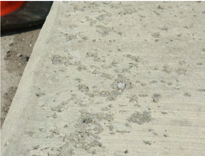
Figure 3. Concrete surface suffering deicer scaling.
