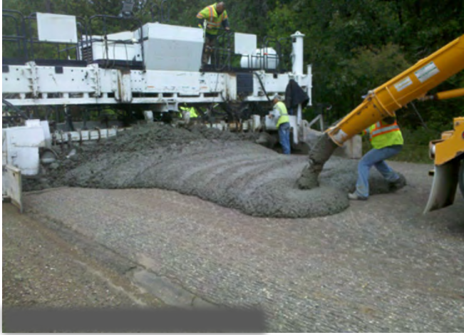
Figure 4. Placement of a 4-inch (102 mm) bonded overlay on a milled asphalt pavement near Devils Lake, ND (NDRMPCA 2015).
