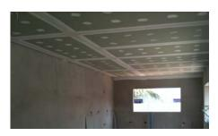
This is a new section requiring floors to be covered with a minimum ½ inch gypsum board or 5/8 inch wood structural panel on the underside. Exceptions are provided for fire sprinklers and certain crawl spaces.
